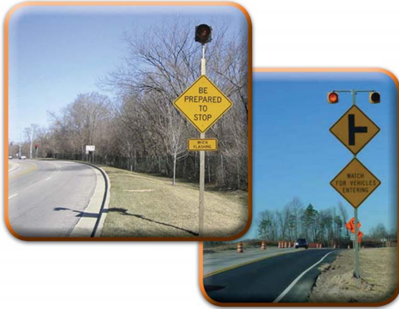
Figure 6.9 Mainline Dynamic Warning Sign
