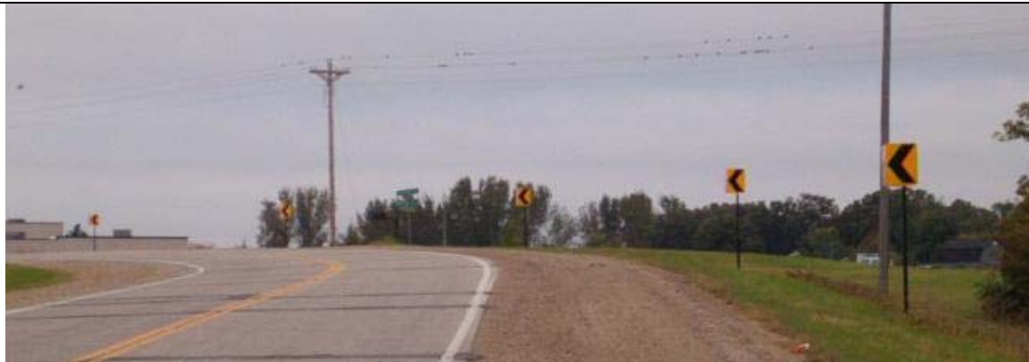
Figure 6.4 Typical Chevron on Curves
