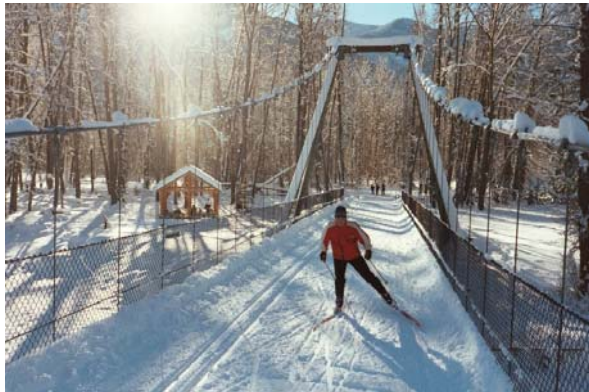
The Suspension Bridge near Mazama, WA.
